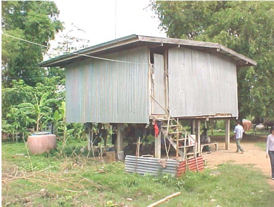
Figure 14: Typical rural dwelling observed. Note the presence of irregular pathways and the need to use stairs to reach elevated living areas. .
